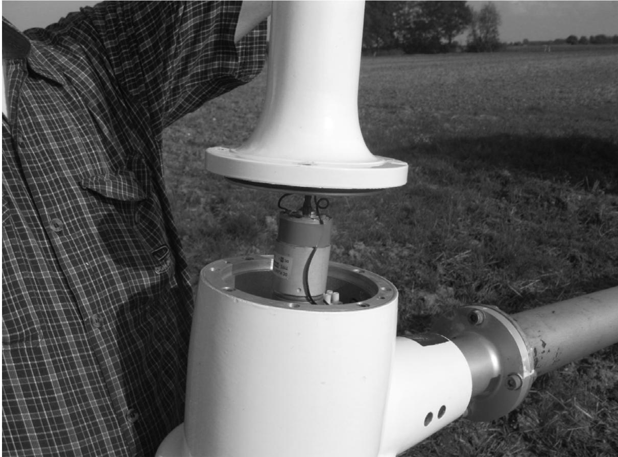
Rotate the housing so that the rear of the housing (the wind vane attachment point) is facing upwards as shown in the above picture. Orientate the wind vane (so that it will point upwards when the generator is raised into position), align the screw holes, and then carefully slide the wind vane onto the housing support flange.
