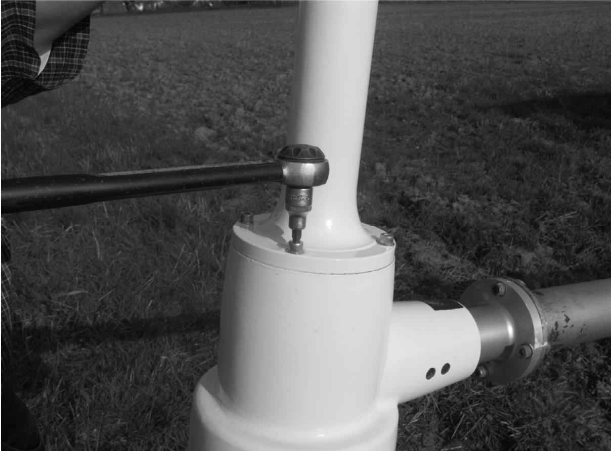
Place one each 8.5mm washer on the four M8 x 50 hexagon screws and inset into the four flange holes. Ensure each of the four screws are installed and hand tight prior to final torqueing. To ensure proper seating of the O-ring seal, tighten the screw alternately a half turn each until snug, then torque to 25 Nm (SAE 18.4 foot-pounds).
